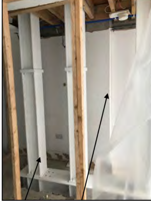
Props & failed steel column
