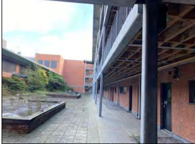
Access via courtyard to apartment 309
