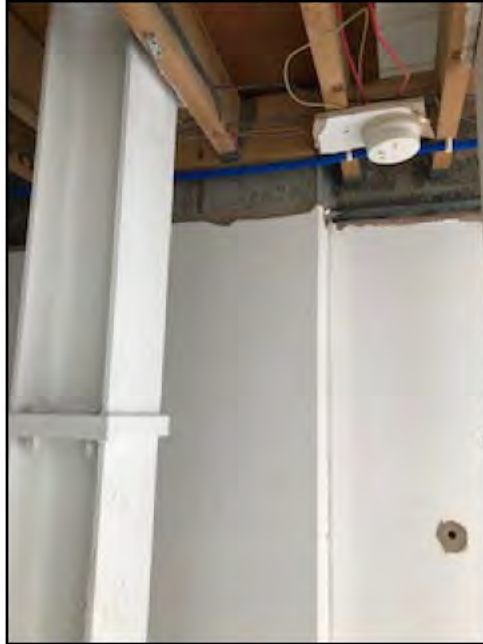
Props & failed steel column
